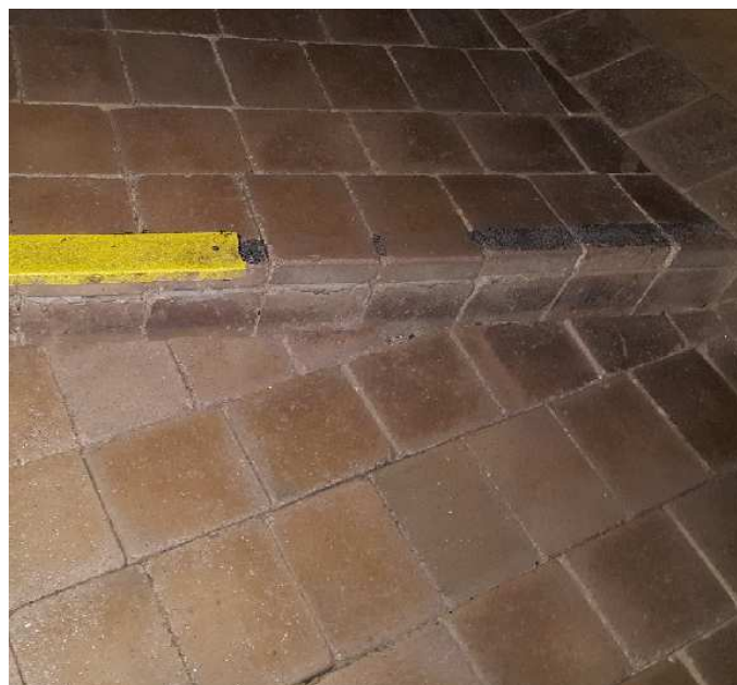
One of the missing stair tread safety strips
